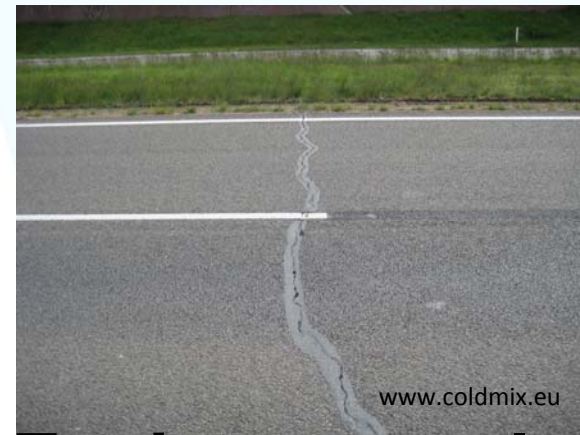
Environmental Related Cracking
